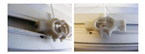
Press on the other side of the aftersales cord guider to instert the legs in the profile. Press one leg at a time.
