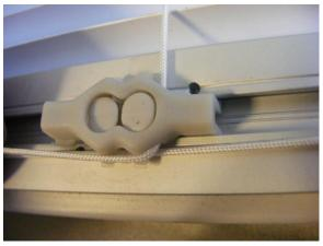
Make sure the cord is guided correctly thrue the aftersales cord guider
